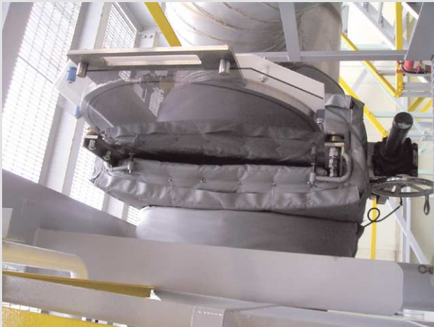
■ 36" compact type blind for isolation
